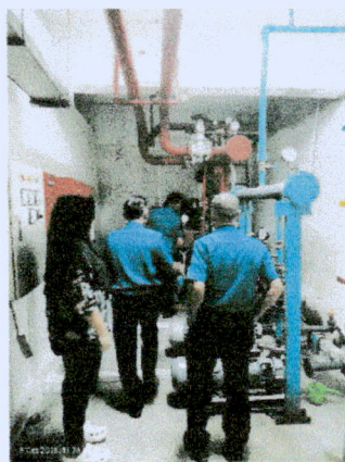
Pengujian Pompa Hydrant
